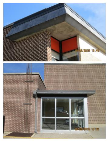
The aluminum storefront appear to be in good condition. However, the painted steel storefronts are faded, stained, with chipped paint and with rusted areas.
