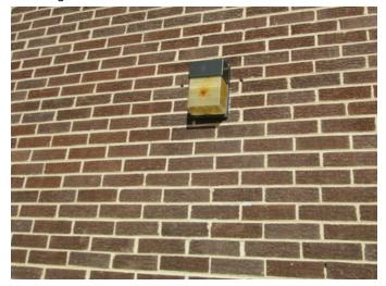
Most of the brick mortar joints appear to be in good condition.
